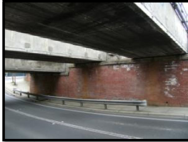
Figure 9: Middle Footscray Rail Bridge
