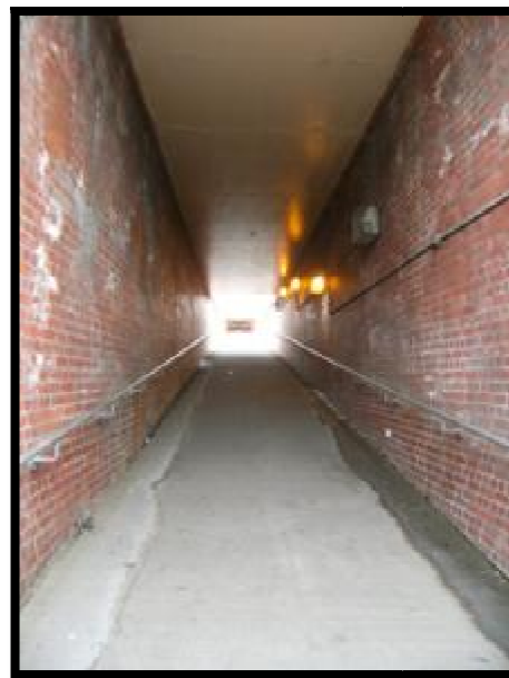
Figure 8: Middle Footscray Station ramp access
