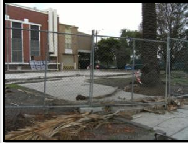
Figure 13: Abandoned building adjacent to Railway Reserve
