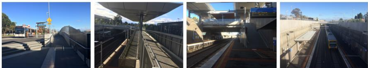
Image 4.4.3 Indicative of footpath condition and Level of Service at Mitcham Station
