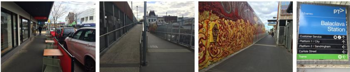
Image 4.1.4 Indicative of footpath condition and Level of Service at Balaclava Station
