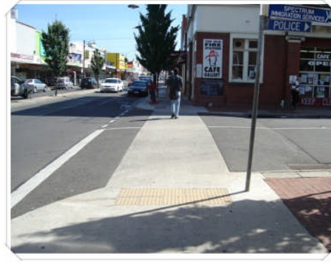
A more appropriate treatment for Exhibition St would be for a raised crossing as in this example from Darebin.
