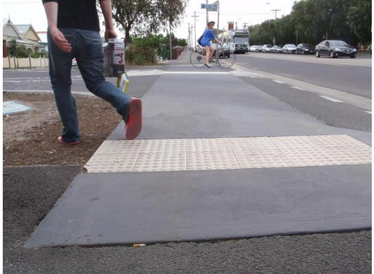
Figure 27 – raised threshold
