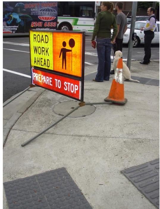
**Figure 9 – a poorly located construction sign presents a trip hazard at the Roslyn/High/Corio Street intersection**
