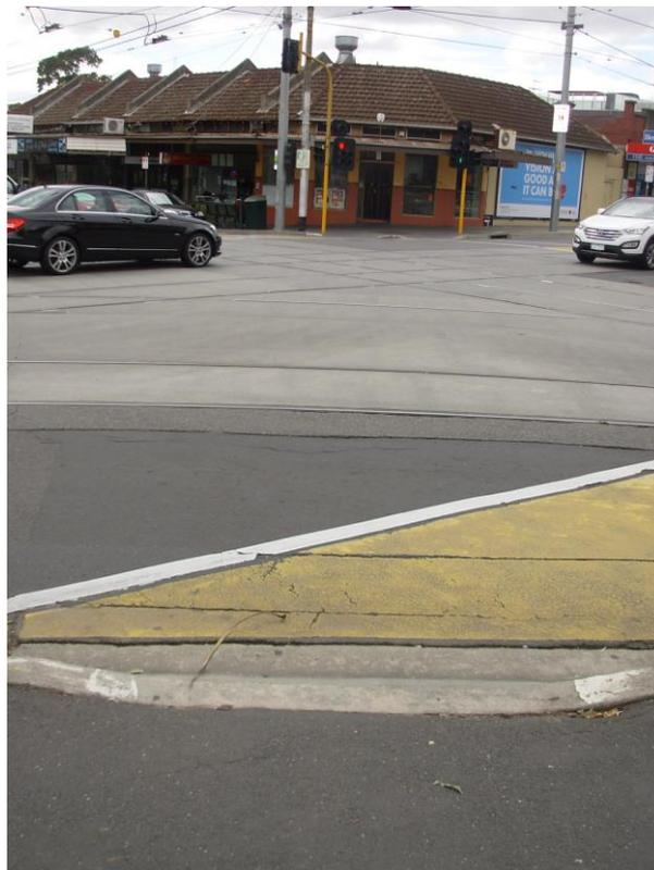
**Figure 26 – kerb ramps oriented towards the centre of the intersection, rather than the direction of the crossing (highlighted in yellow), corner Riversdale and Glenferrie Roads**
