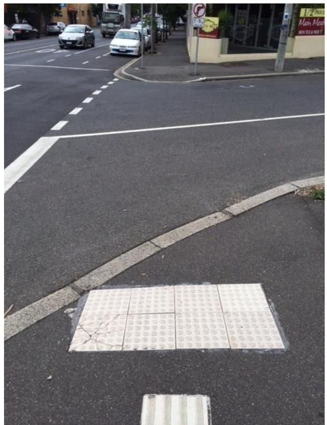
Figure 20 – Poorly configured ramp and absent TGSIs (other side of the road) at Eastwood Street
