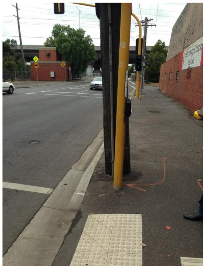
Figure 16 - pole obscuring view to the east at crossing of Macaulay Road, Stubbs Street
