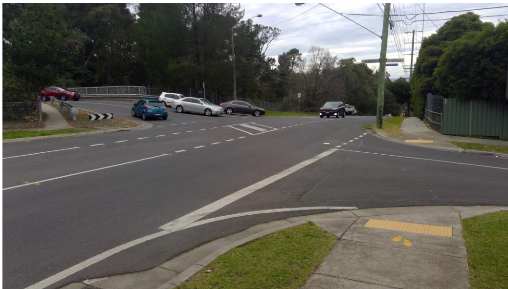
Figure 10 – the intersection of Eastfield Rd (top, all the cars in this photo are on Eastfield Rd), Morinda St (right) and Railway Ave (left).
