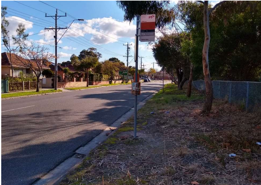
Figure 28 A bus stop adjacent to the train line in Oakleigh South without any footpath
