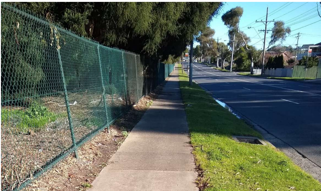
Figure 42 This bus stop in Springvale is adjacent to the Crematorium and there are no kerb ramps or driveways to help people using wheeled devices or with limited mobility to cross the road
