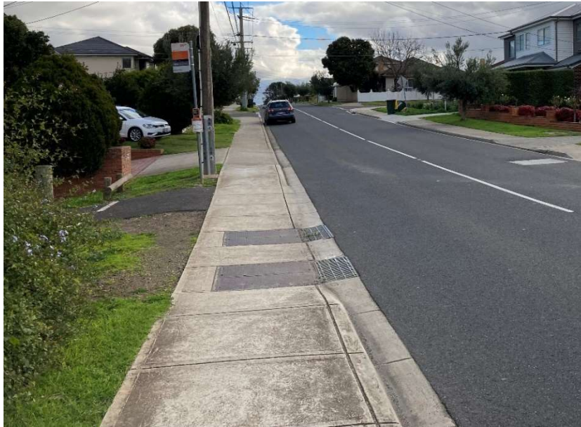
Figure 43 This footpath next to a bus stop in Airport West changes grade at the driveway
