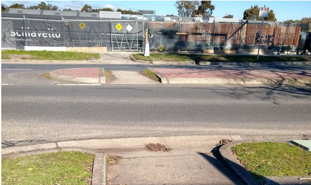
Figure 42 This bus stop in Springvale is adjacent to the Crematorium and there are no kerb ramps or driveways to help people using wheeled devices or with limited mobility to cross the road
