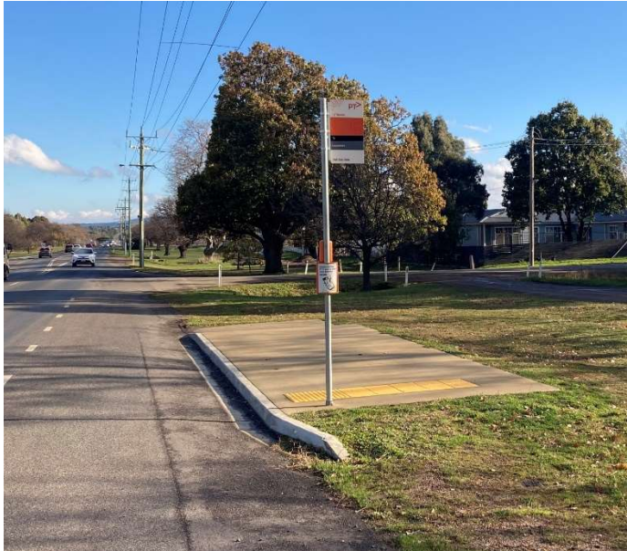
Figure 4 A new bus stop in Riddells Creek which appears to comply with the Standards, but is not accessible to everyone as it has no connecting footpath
