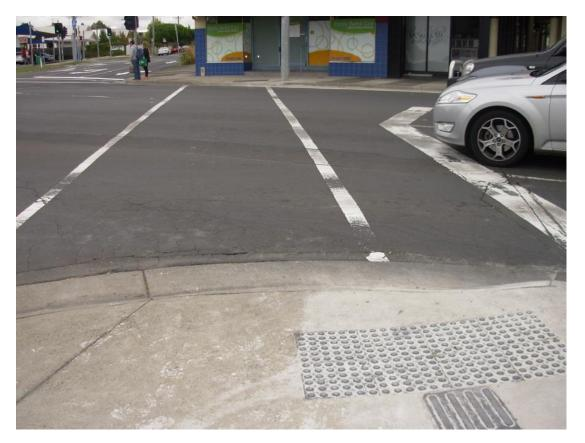
Figure 10 – poorly aligned ramps, TGSI and crossing at the Roslyn/High/Corio street intersection
