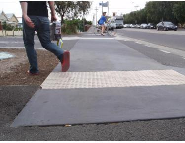
Figure 27 – raised threshold
