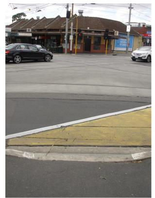
Figure 26 – kerb ramps oriented towards the centre of the intersection, rather than the direction of the crossing (highlighted in yellow), corner Riversdale and Glenferrie Roads
