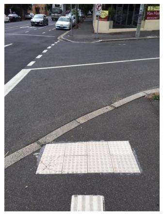
Figure 20 – Poorly configured ramp and absent TGSI (other side of the road) at Eastwood Street
